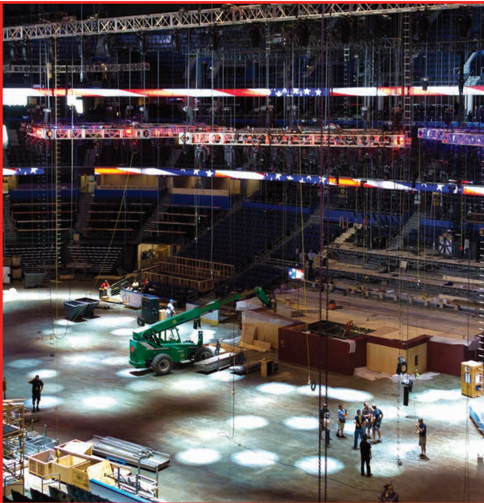
The load-in. The RNC light rig included PRG Best Boys; Philips Vari*Lite VL3000 Spots, VL3500 Spots, and VL3500 Washes; Clay Paky Alpha Spot HPE 700s; and GLP Impressions.
