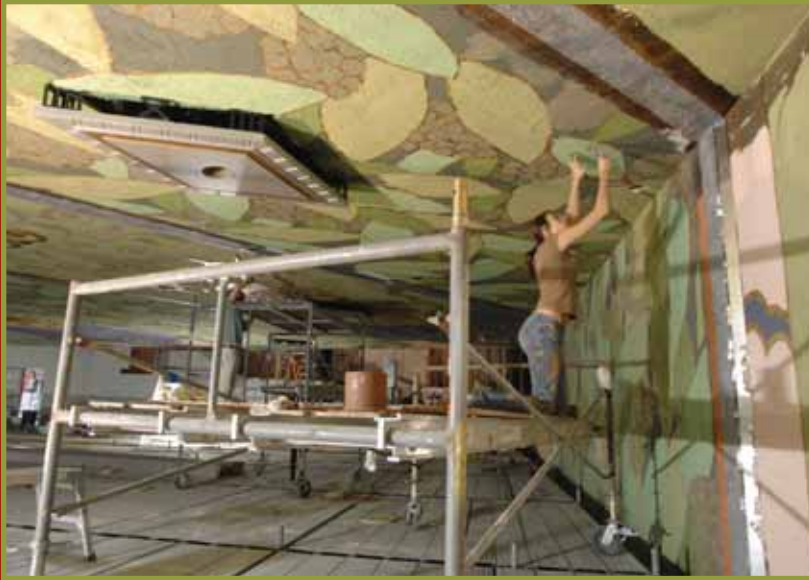
Restoration work focused on all of the theatre's decorative details.
