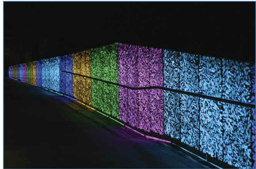
Using Color Kinetics' Light System Manager, every foot of ColorGraze on the bridge's 208' span is individually controlled.
