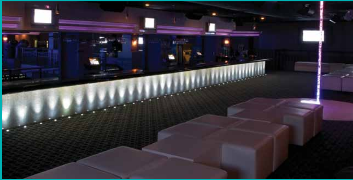
The VIP bar features pearlescent white Italian tile, lit with 40 pieces of ArcSource 1 ten-degree LED units.
