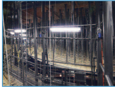
Figure 6: Guide tubes between grid and plaster ceiling.
