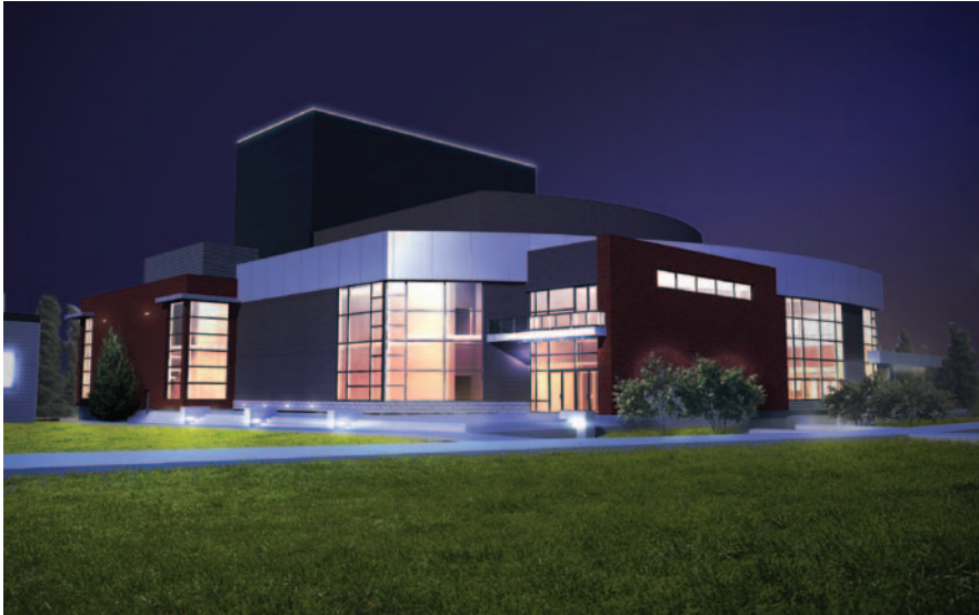
The Jeanne & Peter Lougheed Performing Arts Centre in Camrose, Alberta features all LED lighting fixtures powered by a solar panel clad fly-tower.
