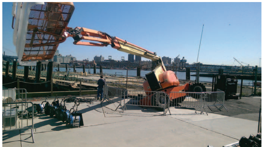
Determining that the work surface can support the weight of the MEWP is just one of the required steps in the Risk Assessment of the work location.
