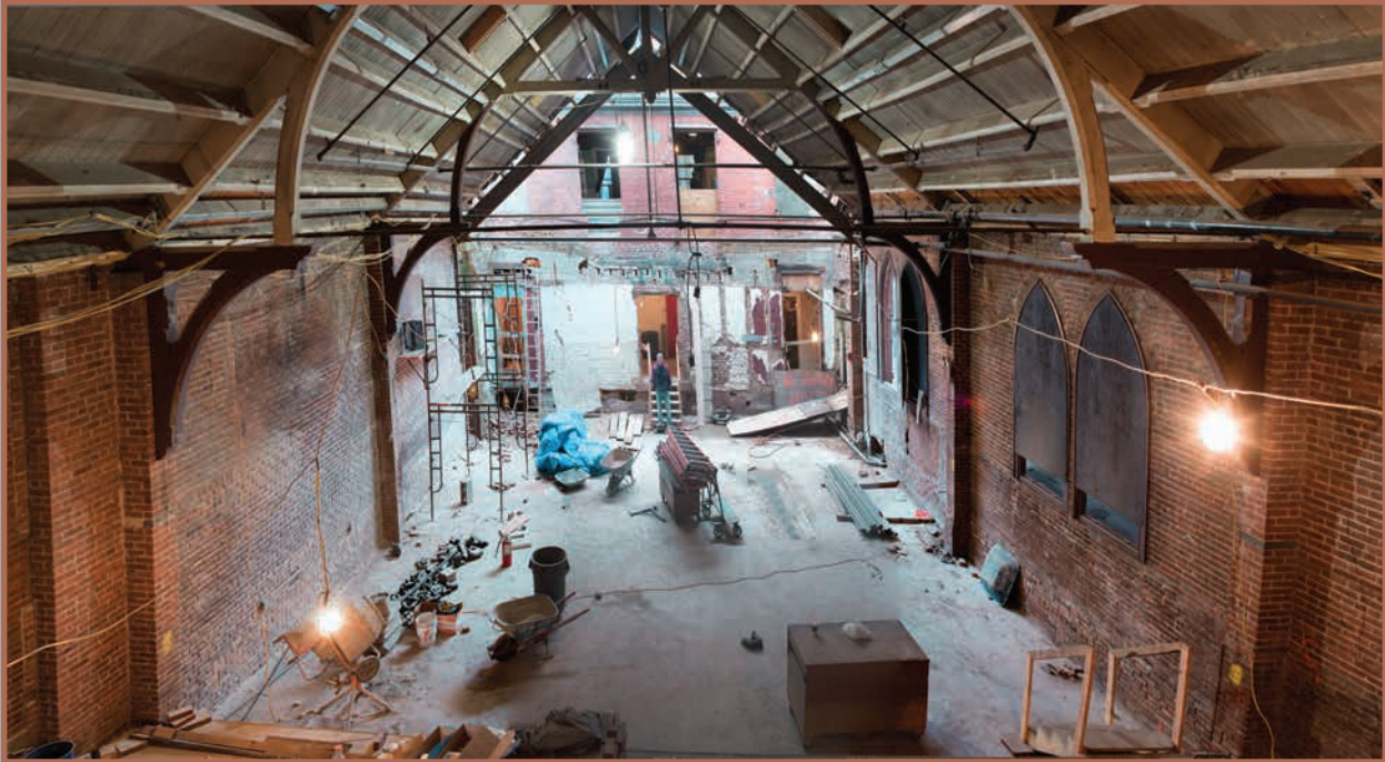
The back wall of the theatre was moved 9', which also required the removal of a supplementary building that stood in the way.
