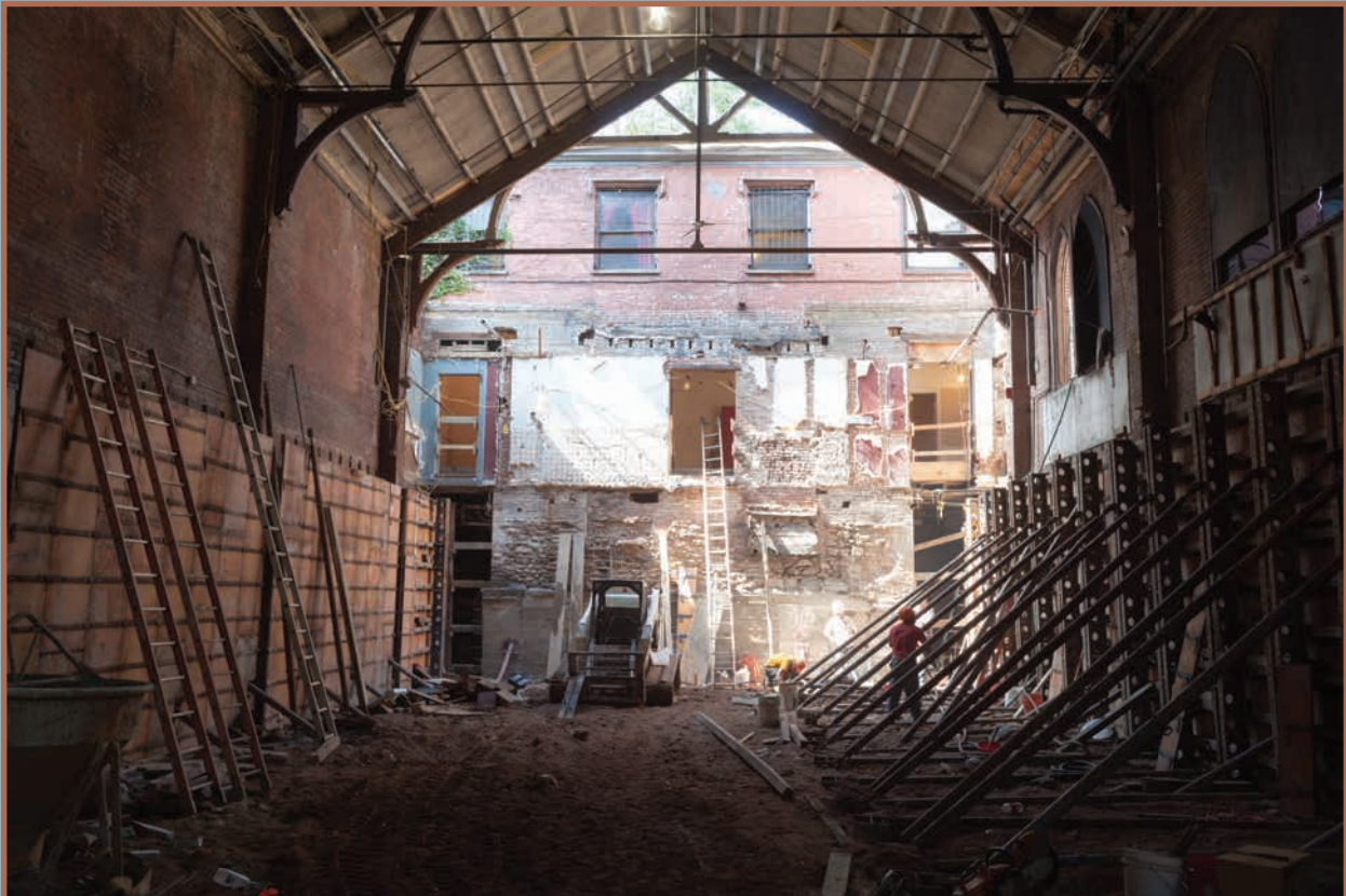
The back wall of the theatre was moved 9', which also required the removal of a supplementary building that stood in the way.
