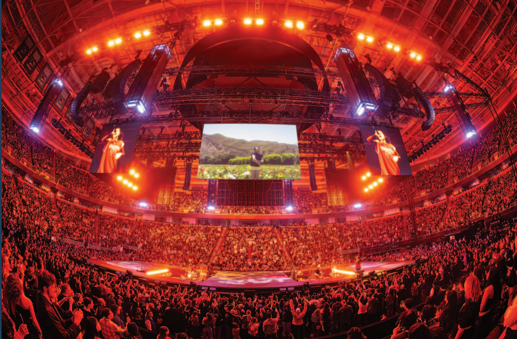
Above: In the PA are eight clusters of 20-deep Cohesion CO10s, and two hangs of eight-deep CO10s on the far sides of the stage to cover the floor on the goal ends. There are four end-fire arrays consisting of two hangs of three CP218s each. On the ground are 12 clusters of three CP218s in cardioid, plus 24 CO8s for front fills.
