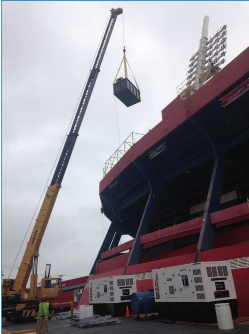
There were no elevators, so a crane was used to place the Vari-Lites, cabling, and power distros onto the scaffold on the upper bowl and in the bleachers.
