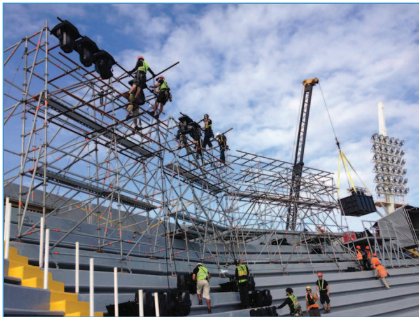
Eight large scaffold towers were built in the upper seating bowl, each of which housed 36 of the new Philips Vari*Lite VL4000 Spots and 36 VL3500 Wash or VL3500 Wash FX fixtures.
