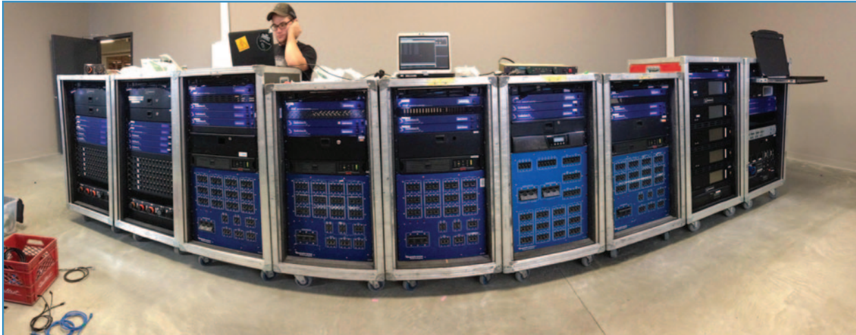
Solotech assembled and tested nine racks of data distribution, including MA Lighting nodes, 12 ELC dmXLAN Switch8GB switches and eight ELC dmXLAN Switch8LX Fast Ethernet switches, plus 24 ELC dmXLAN Node 8S gateways.
