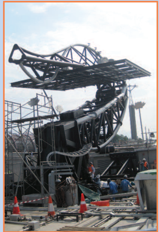
A crane's body, installed on the barge at Sentosa.
