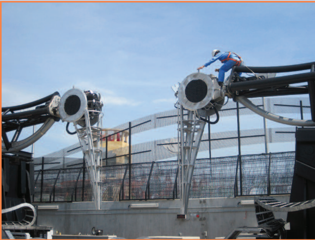
A worker tinkers with one of the crane's eyes.
