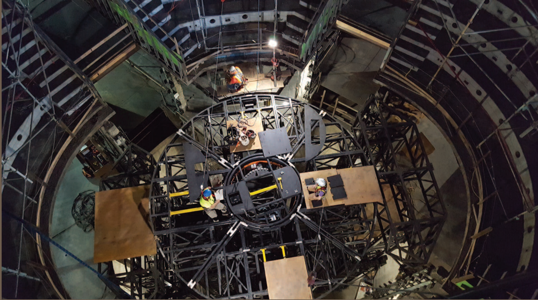
Installation of the center lift.
