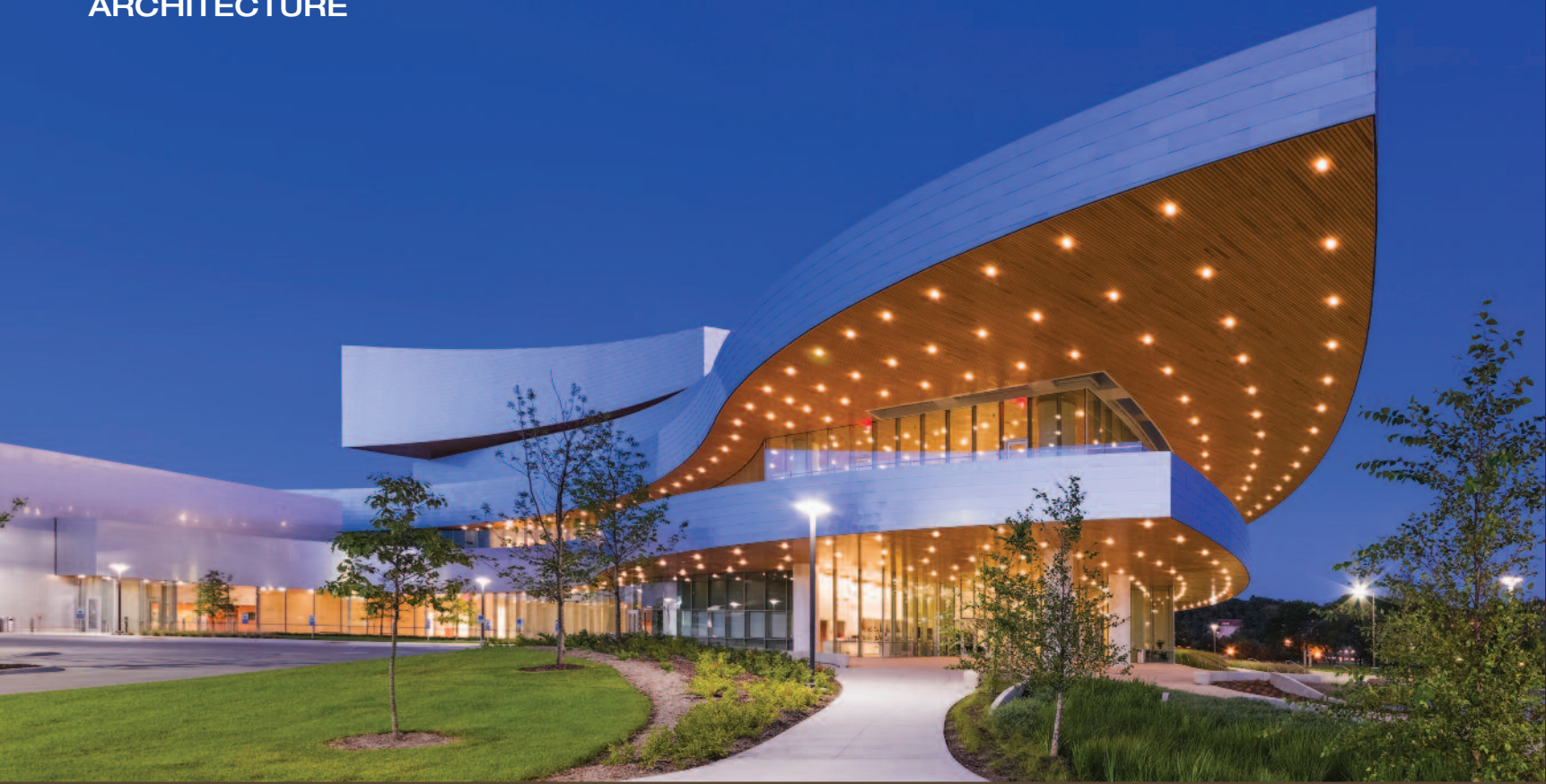
Above: The building's outer curves are covered in stainless steel with a brushed angel-hair finish, and lined underneath with cypress wood. Opposite: The spacious, light-filled lobby reflects the architect's mandate to create a more transparent building.
