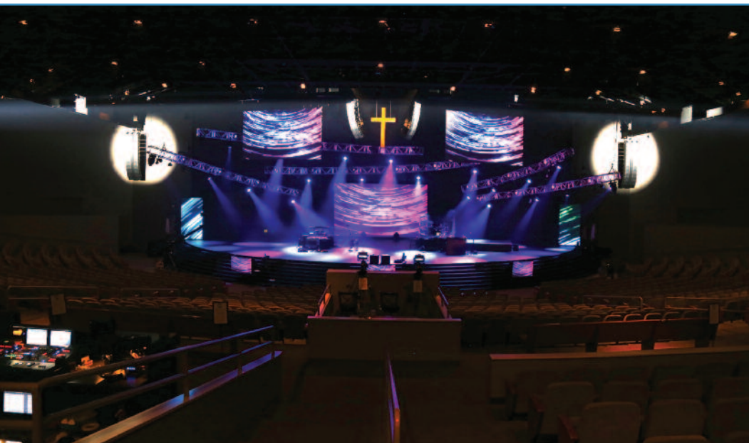
Full AVL configuration is visible in this photo, with line arrays, LED screens, RP screen, and LCD displays.
