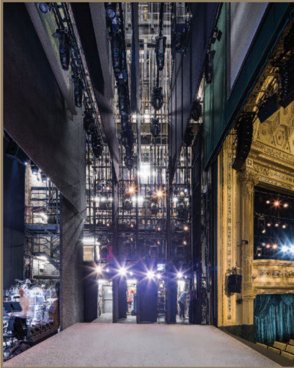
Weihs installed the double-purchase counterweight line set system.
