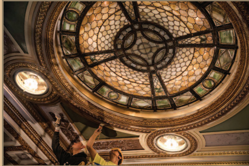
Each piece of glass in the domes was removed and cleaned by hand.
