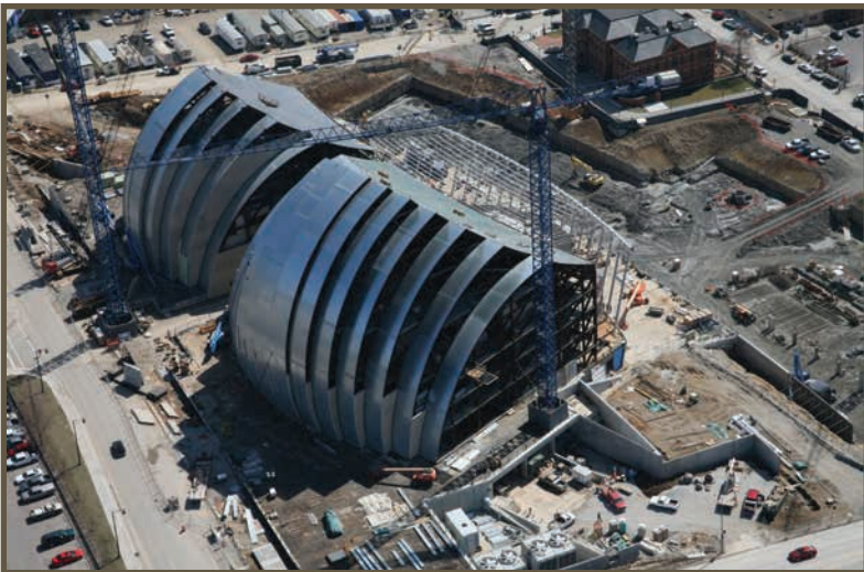
The building, consisting of two mounds of steel-sheathed, arched segments, under construction.
