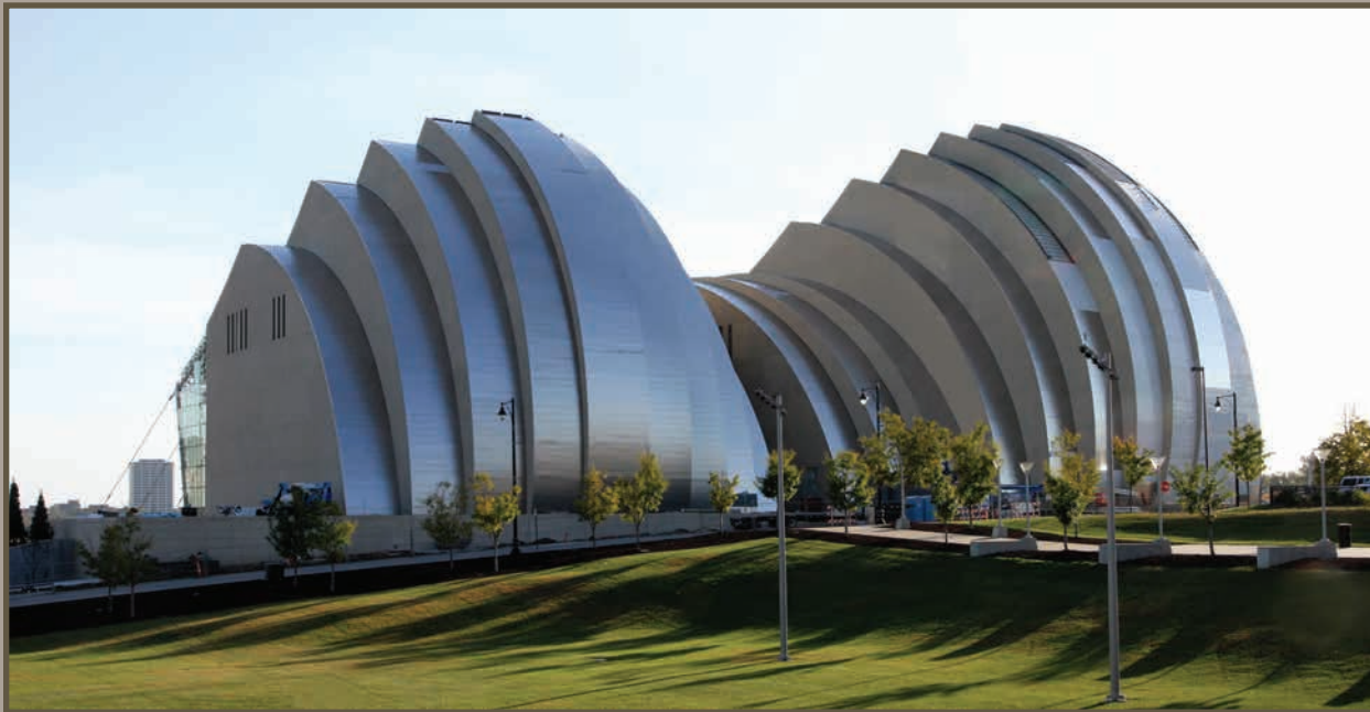
On its hill, the dramatic structure of concrete, steel, and glass is surrounded by five acres of green space.
