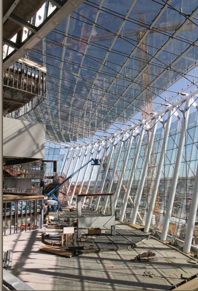
The Brandmeyer Great Hall under construction.
