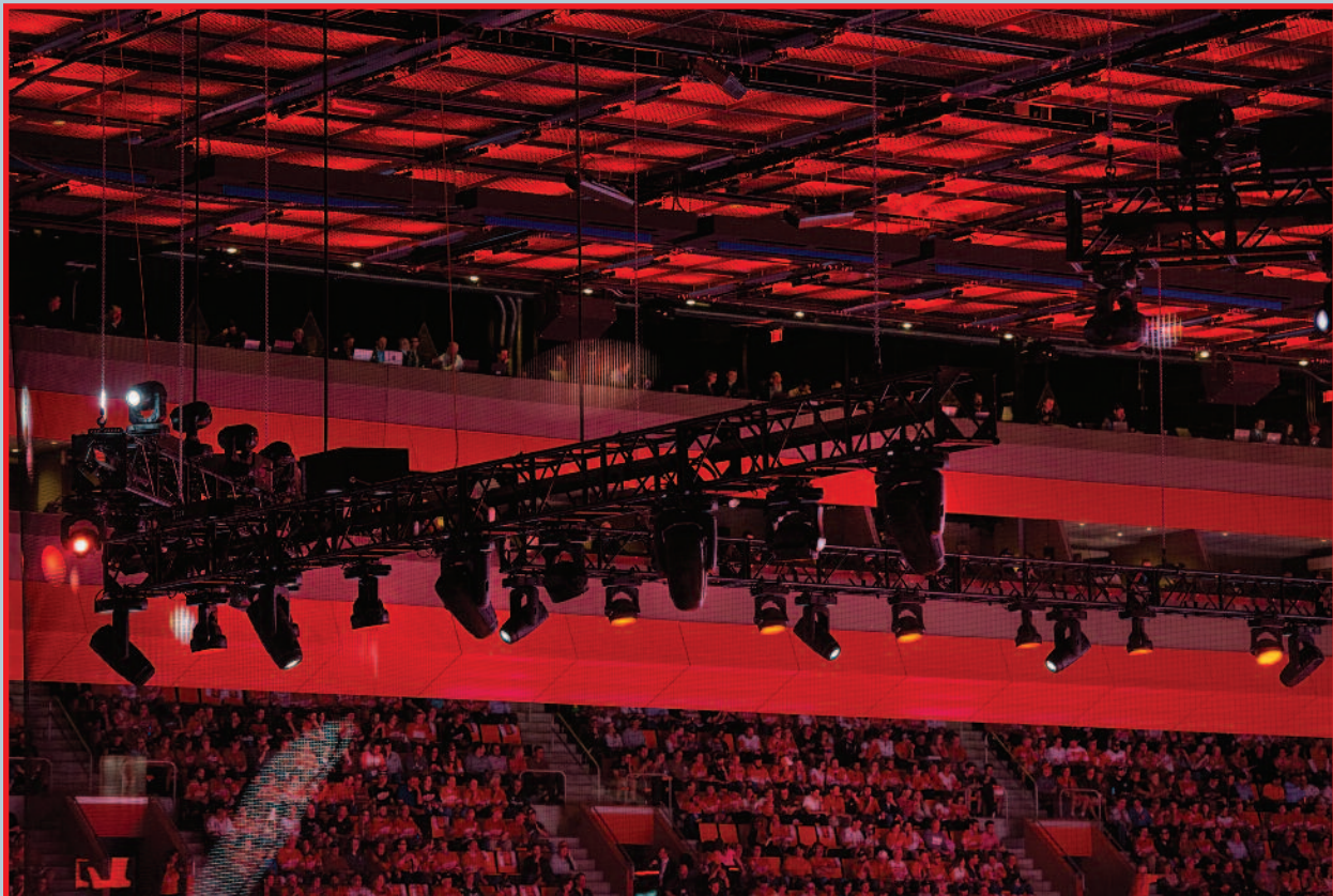
Rigging of the trusses, handled by ARS, includes variable-speed hoists.
