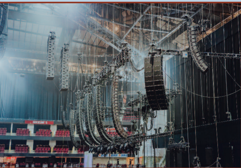
The Lorde L-Acoustic PA hang can include up to 13 separate hangs, including some over the seats.
