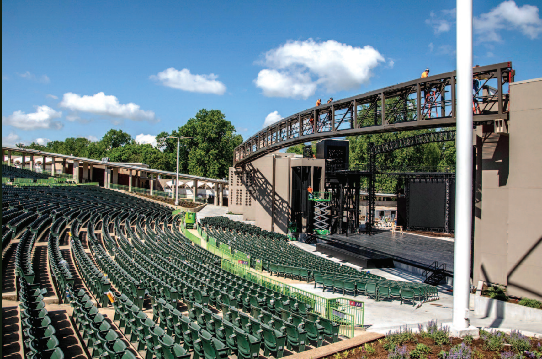
A new and enlarged lighting bridge, made of structural steel, features an integrated walkway that accommodates enhanced lighting configurations.
