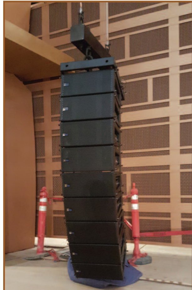
One of the theatre’s Meyer Sound MINA line arrays.
