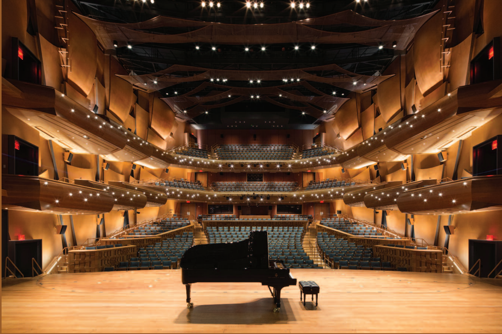
A major design feature of Julianne Argyros Orchestra Hall is the sidewalls, which feature heavy construction and diffusive elements specified by Toyota.
