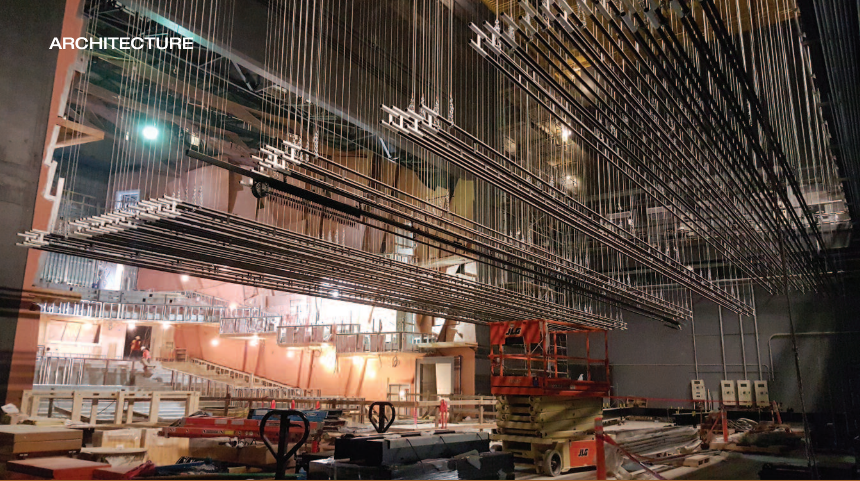
The rigging system, seen during installation.
