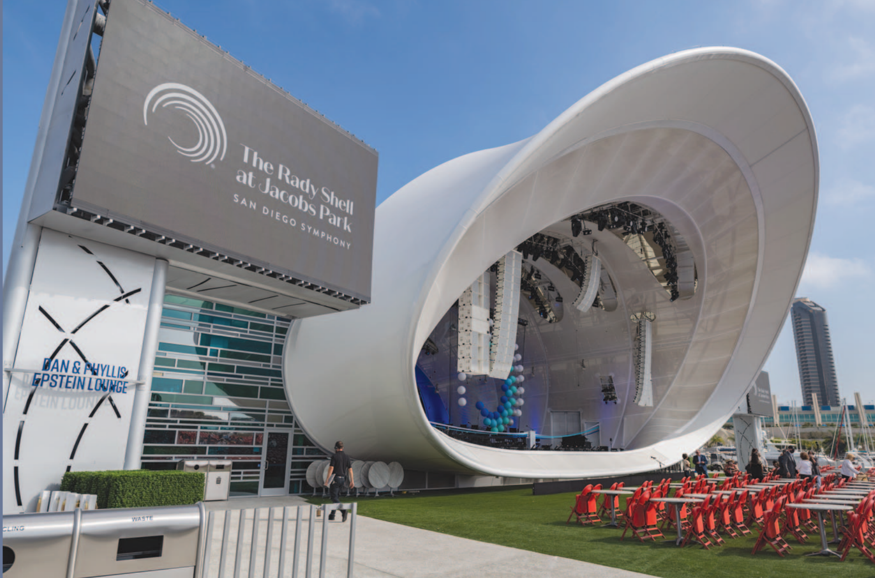
The Rady Shell stage features concentric widening oval rings as its canopy, a structure that reaches a height of 57' and a width of 92' at the front of the stage, which spans 4,800 sq. ft.
