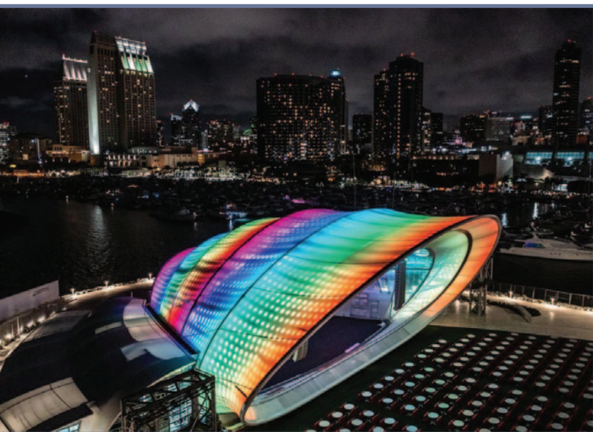
The shell structure also features 3,386 individually controllable Traxon LED light nodes for artist-programmed light shows.
