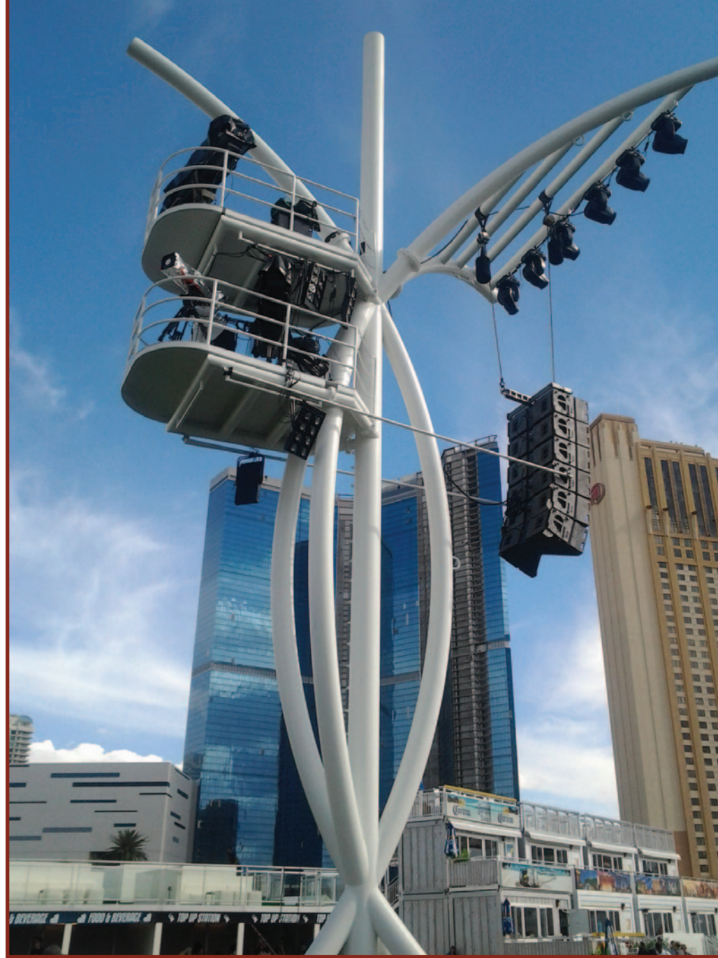
The permanent delay towers, stacked with PA and lighting.
