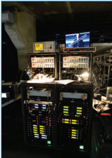
Wireless receiver racks in the RF area.
