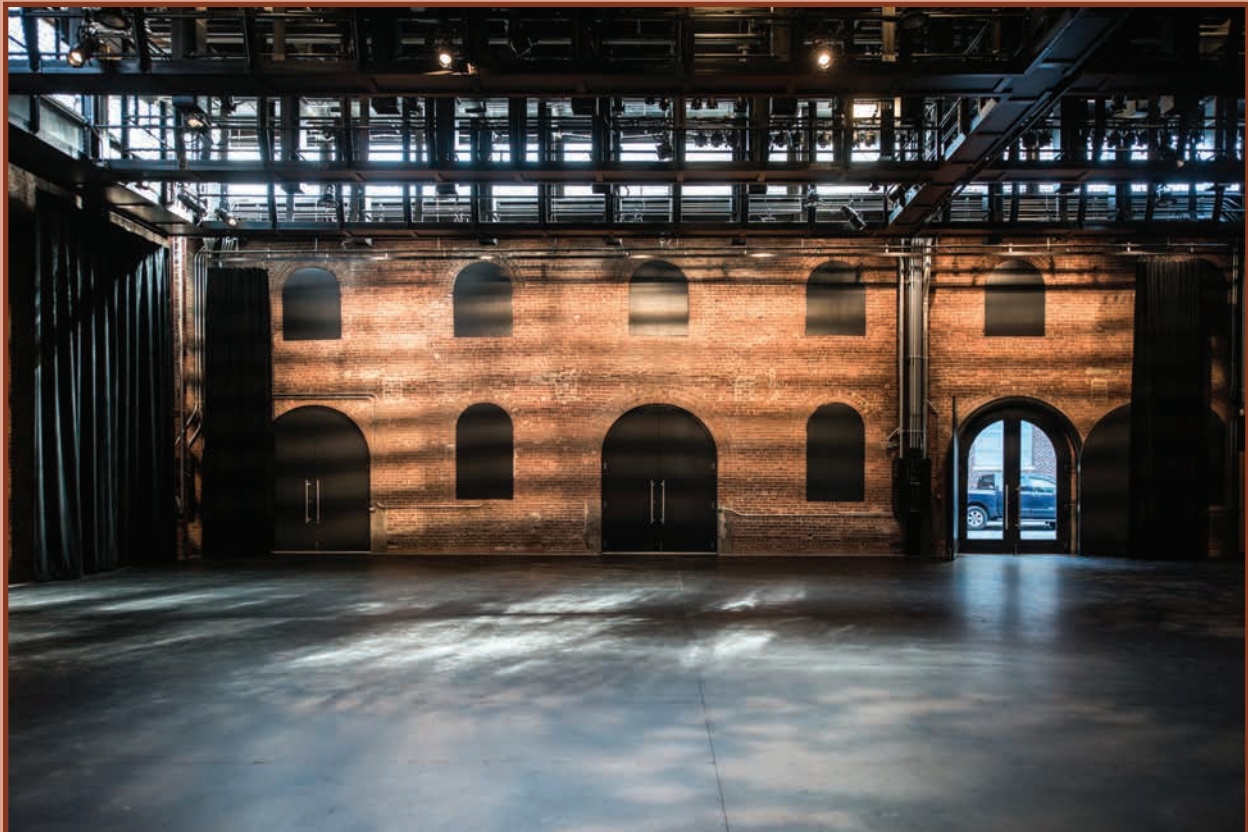
The building's original windows were restored; those in the theatre are covered with solid acoustic doors.
