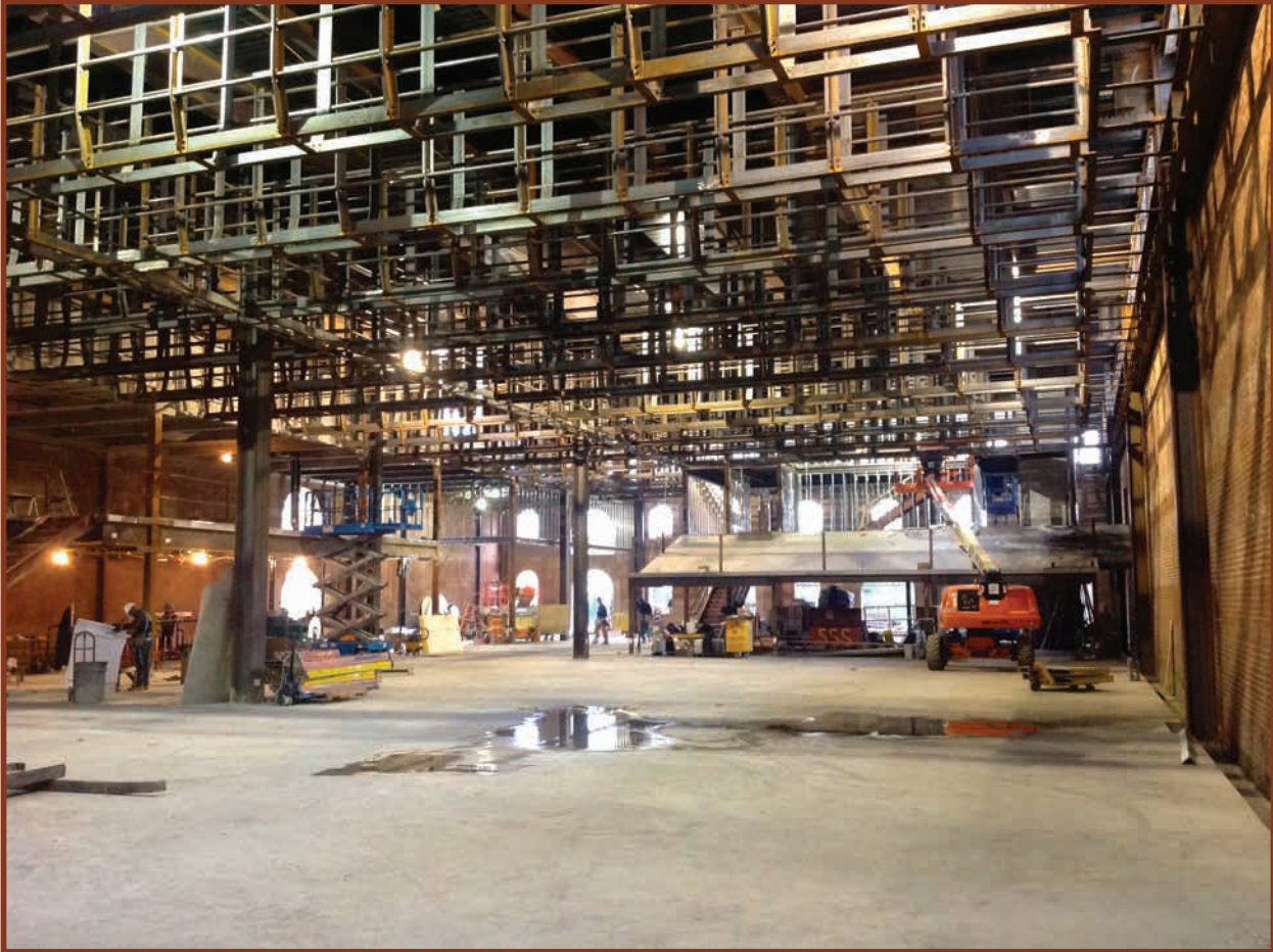
An interior view of construction. The theatre's support columns are next to, but do not touch, the original walls.
