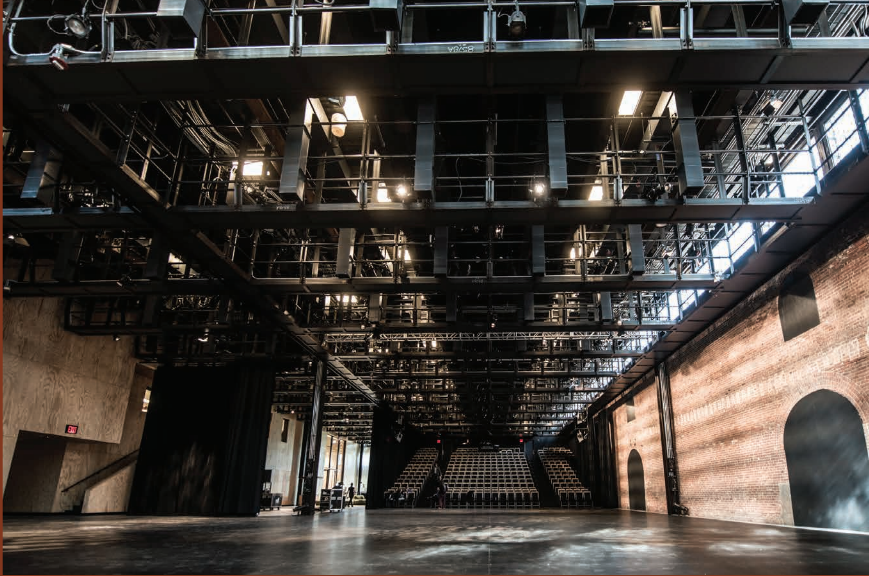
The catwalks are placed every 10' and extend into the lobby.
