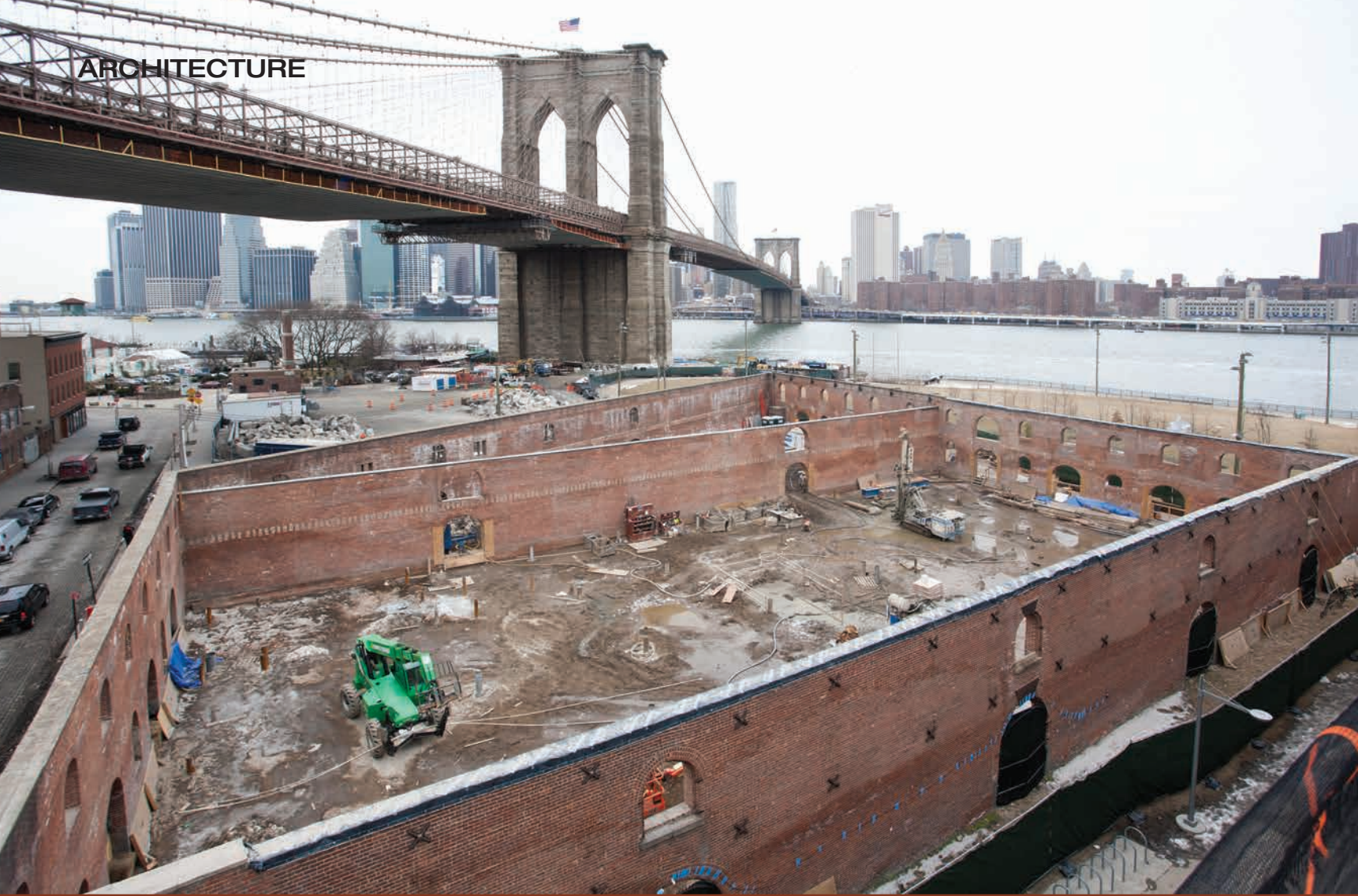
The theatre under construction; great care was taken to ensure the integrity of the original warehouse structure.
