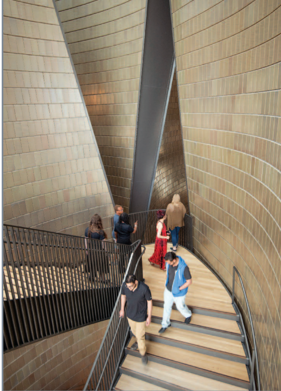
The interior and exterior walls are clad in 220,000 glazed terra cotta industrial tiles finished in semi-matte graphite and bronze.
