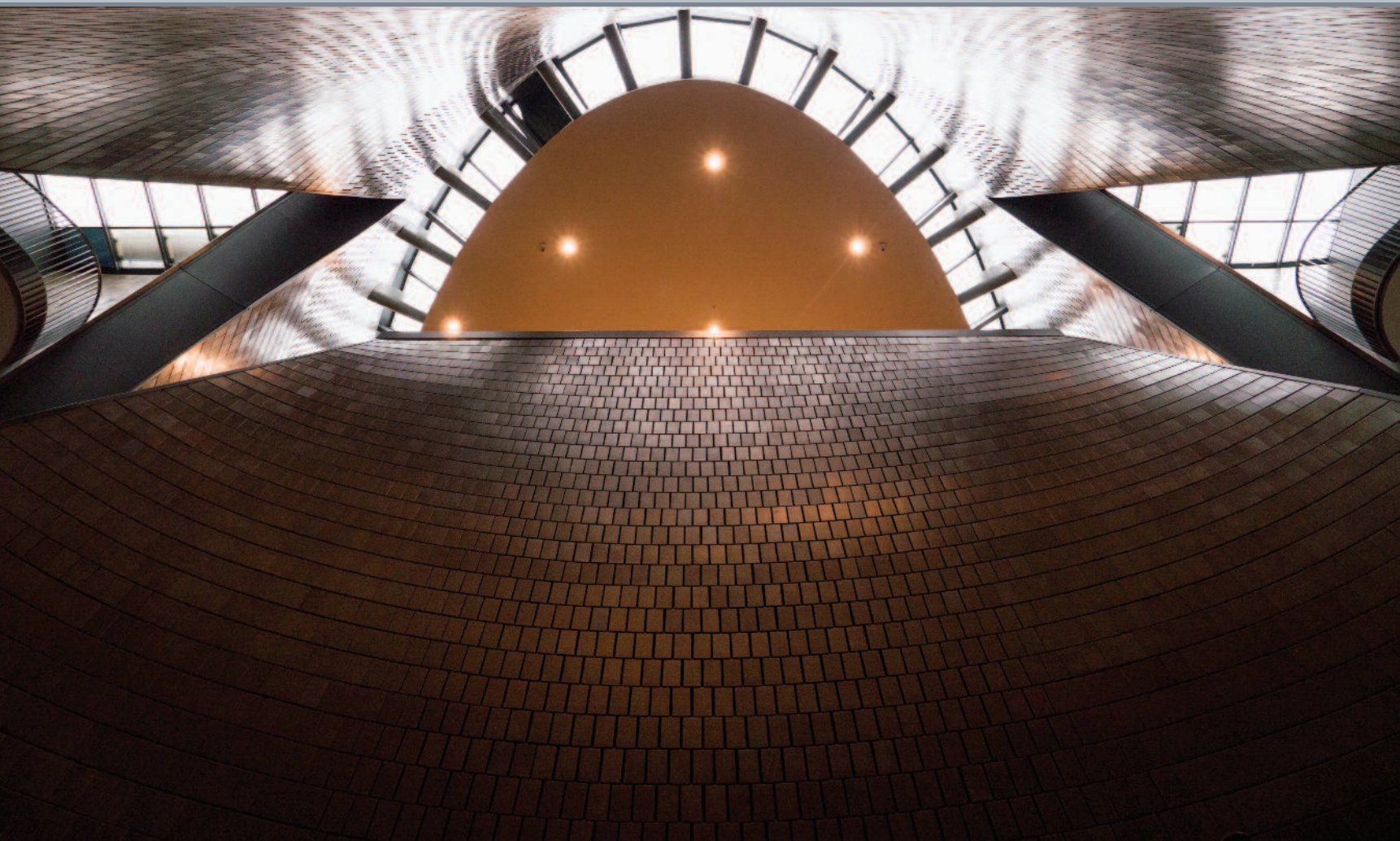
A wall of glazed ceramic tiles, incorporating acoustically tuned slat absorbers, soars upward to a fifth-floor open gallery with an absorptive plaster ceiling that behaves acoustically like open sky; in that event, sound is not reflected back down to the lower levels.
