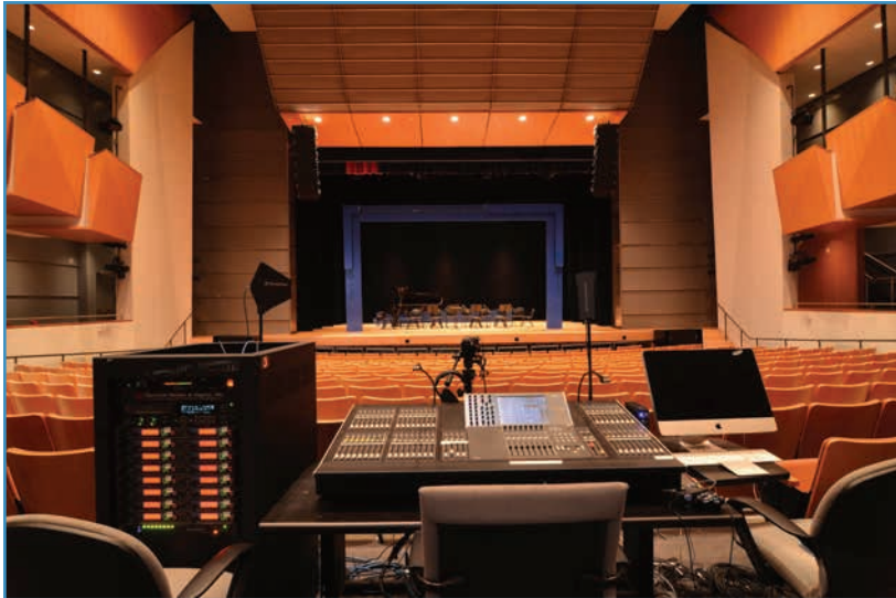
The front-of-house position with the installed Yamaha M7CL-48 console.
