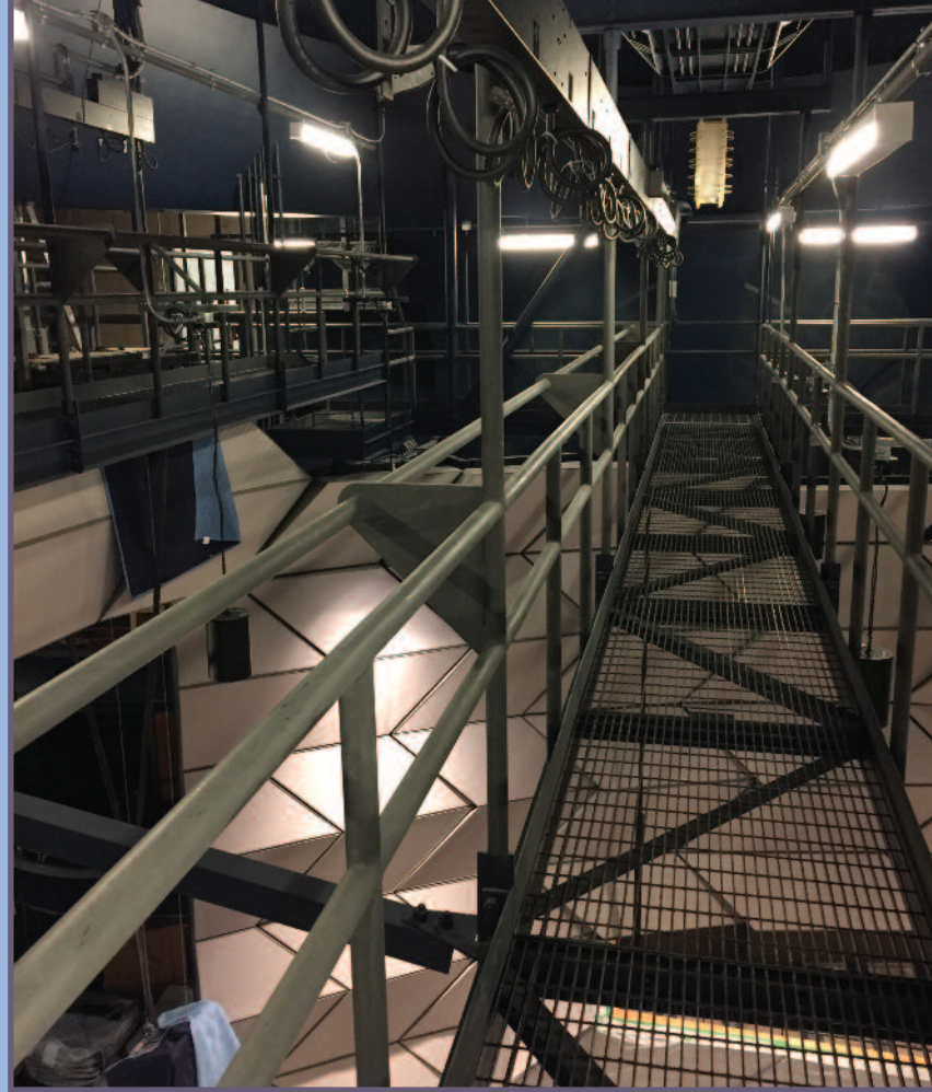
Above: The new front-of-house catwalk in the Lyric. Below: A new tension wire grid runs over the Greenwin stage.
