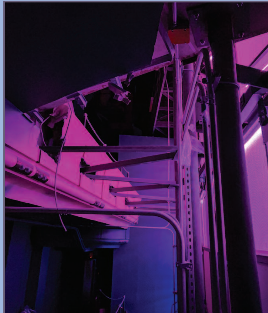
Below: Part of the infrastructure tying the inner shell of the Lyric to the existing structure of the Main Stage.
