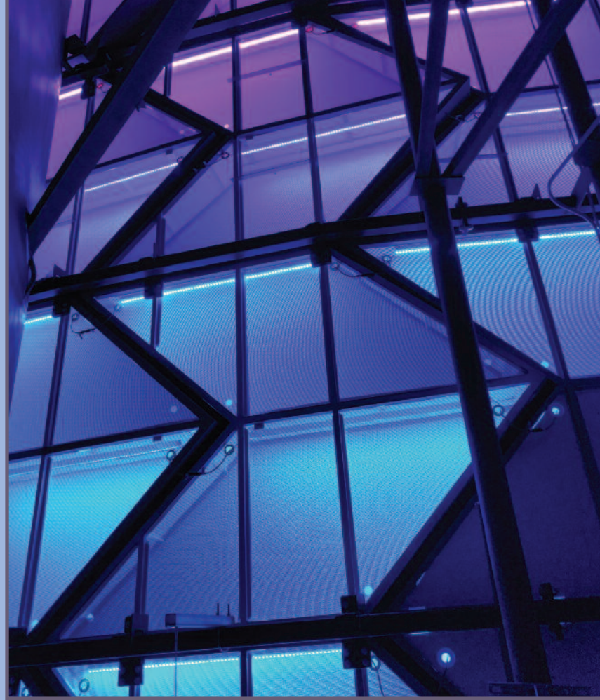
Below: Part of the infrastructure tying the inner shell of the Lyric to the existing structure of the Main Stage.
