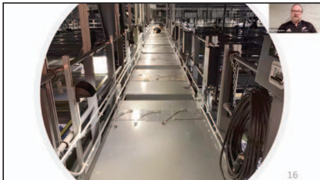
Catwalks provide solid access to the tension grid at the Chase Center Arena in San Francisco.
