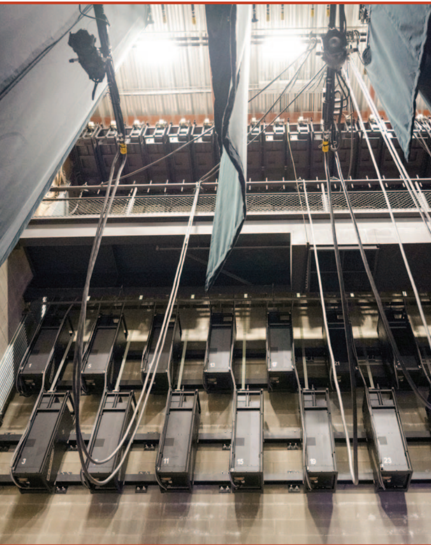
Prodigy EXO motorized hoists automate the overhead stage rigging for lighting, scenery, drapes, and related theatrical equipment.
